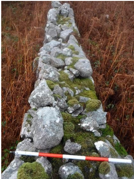
Plate 13.33 - TB 11 showing construction of drystone granite wall
